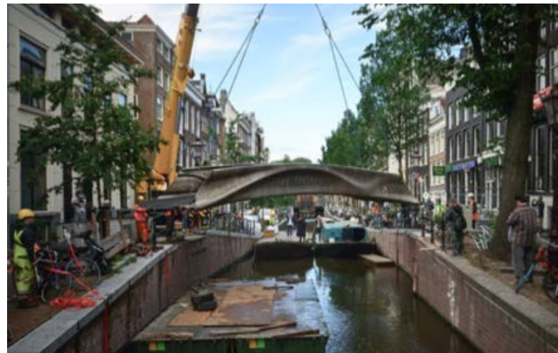
Fig. 3. The M3XD bridge being installed.
