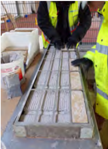
Above: Brick slips being applied to gravel boards
