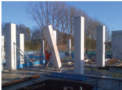
Efficient construction of The Edge comprised prefabricated building assembled at site. Illustration: PLP Architecture
