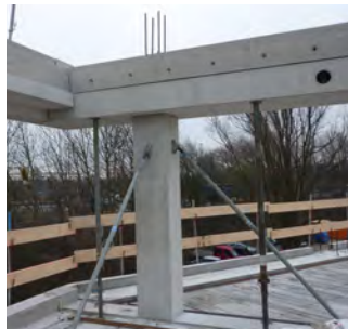
Efficient construction of The Edge comprised prefabricated building assembled at site. Illustration: PLP Architecture
